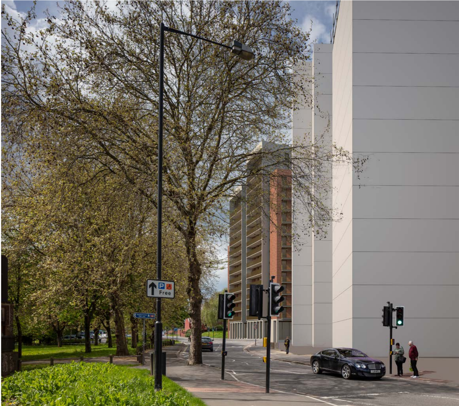
CGI - View from Malago Road as you would approach the scheme from the city
